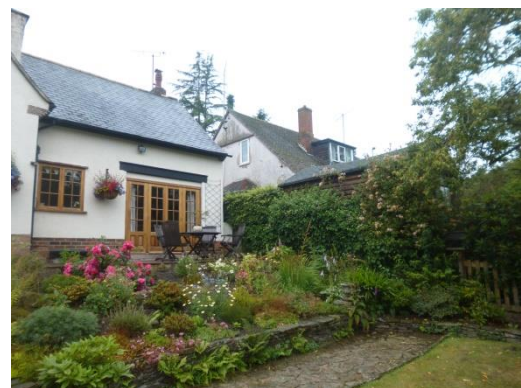
Photo taken facing south west towards No 17 and No 19
